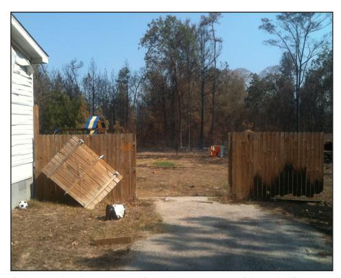
This home on the Riley Road Fire didn't ignite because a portion of the attached fence was removed, preventing the fire from spreading to the house. Many other homes in the fire's path weren't as fortunate.
