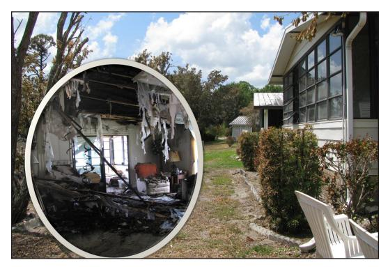
Embers from a nearby fire gained access to this home's interior, igniting it and causing significant damage.
