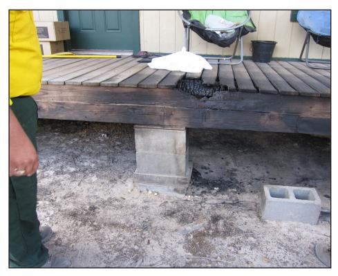
The porch of this home on the Dyer Mill Fire was ignited by embers that were spread by strong winds. Fortunately, a fire engine was stationed near the home and firefighters were able to extinguish the blaze before it spread to the house.
