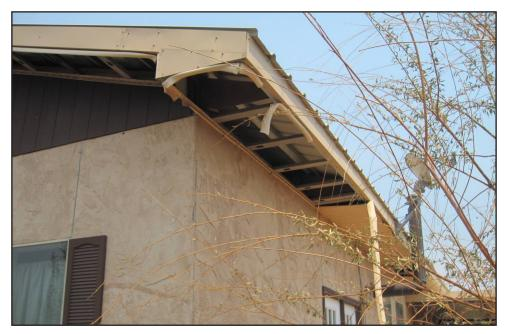
Combustible soffits can melt or ignite, giving embers access to an attic. Once inside, the embers can go undetected until it is too late to save the home.
